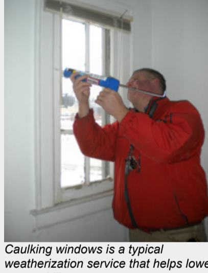
Caulking windows is a typical weatherization service that helps lower energy bills.
